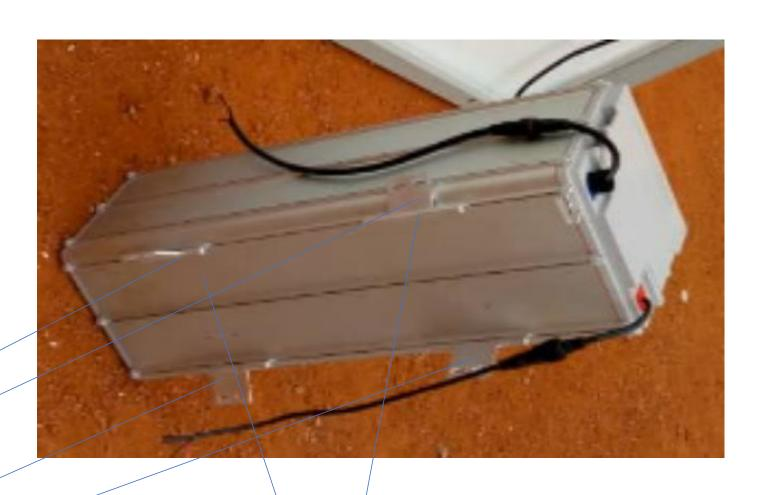
The distance of two tabs can be adjusted based on solar panel bracket hole distance.
