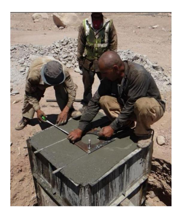
Bolts Size should be the same as Pole Flange Screws
